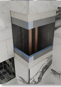
Multiboard pipe boxing can be stacked up to the necessary height, just put a bead of Marmox MSP360 where the Multiboard meets.
